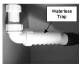
escape into the RV interior. The waterless trap can be unscrewed from the water lines. A label has been placed near the location of the waste valve that reads as follows:
